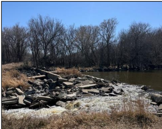
Figure 4.5: Dam near Redfield Cemetery.
