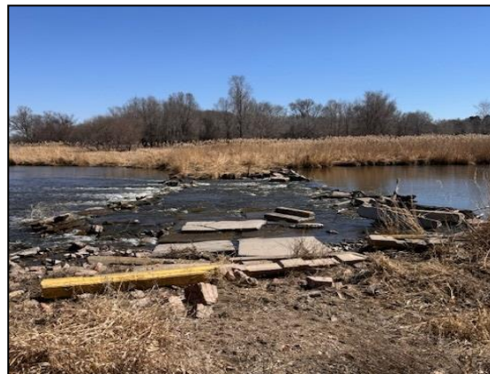
Figure 4.6: Dam near SDDC in Redfield.
